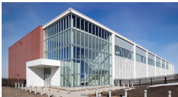
Illinois Petascale Computing Facility
